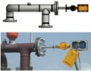
Original OWD installation and spool design / actual unit during install.
